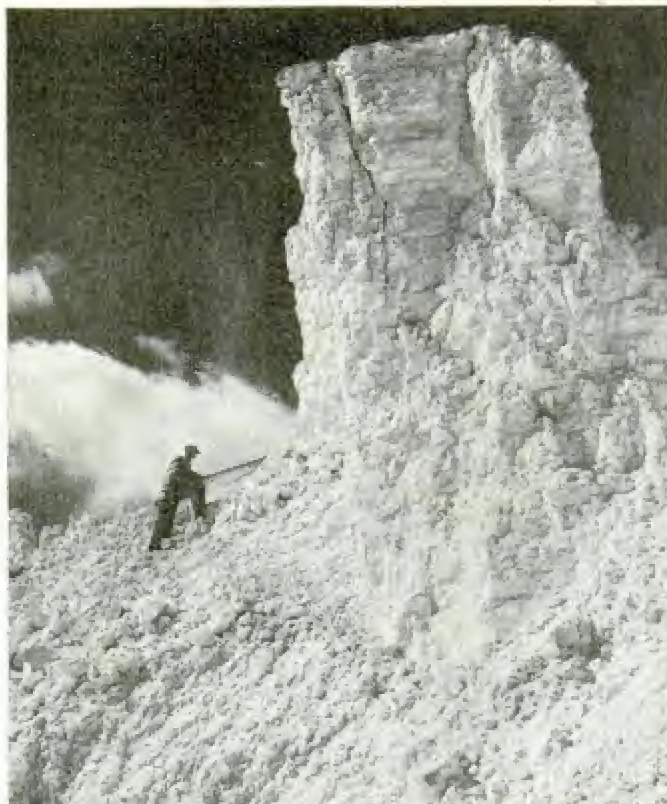
Drilling a hole for a charge of explosive that will break up the storage pile so it can be loaded in cars by huge shovels. Below, a golden stream of sulphur dust flows through spout from weigh house to load a Mississippi River barge in Louisiana
